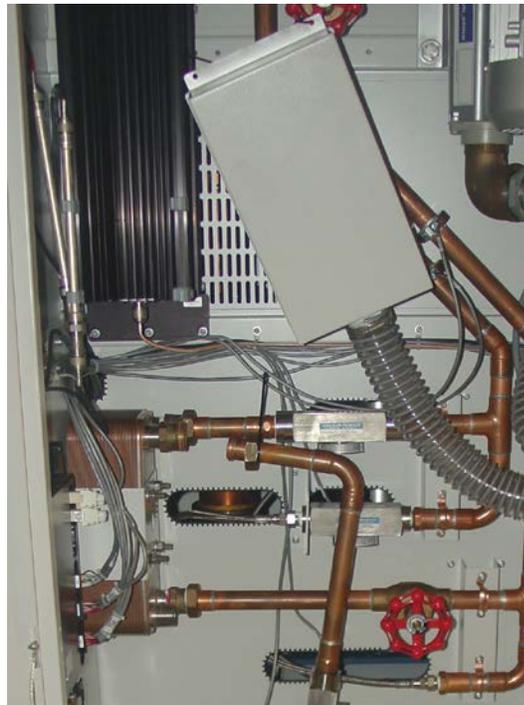
Cavity Blower Air Filter, RF filter and Upper HX pipe Tied Off
