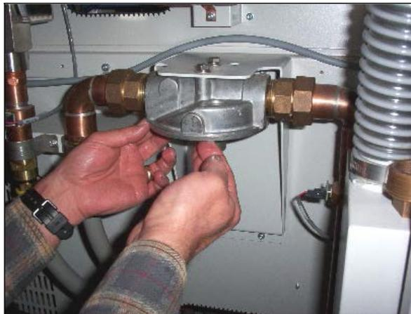
8. Install new filter by turning it clockwise onto fitting. Be careful to not cross-thread the filter.
