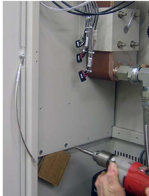
9. Drill the first two (2) holes using the counterbore bit, as illustrated above, removing paint from the panel. Carefully vacuum any and all metal shavings that were generated.
