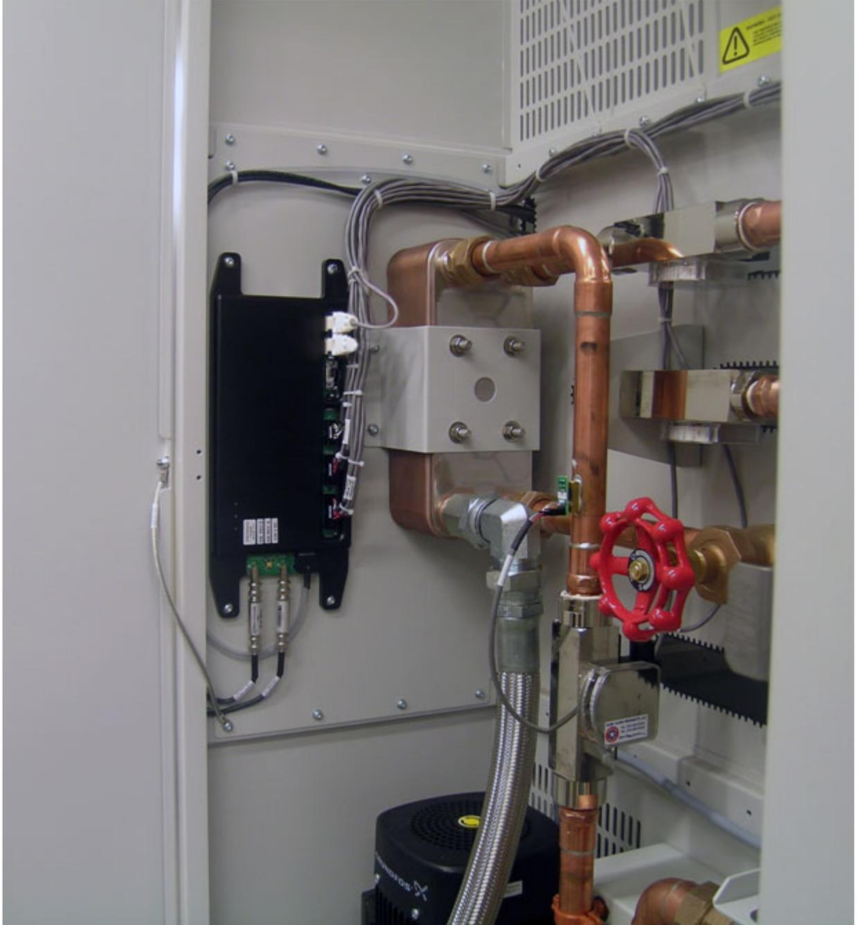
Modified IOT/C-I/O Module installed
