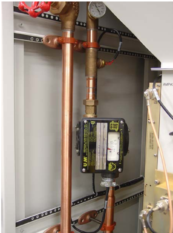
Obsolete Piston-Type Flow Monitor
