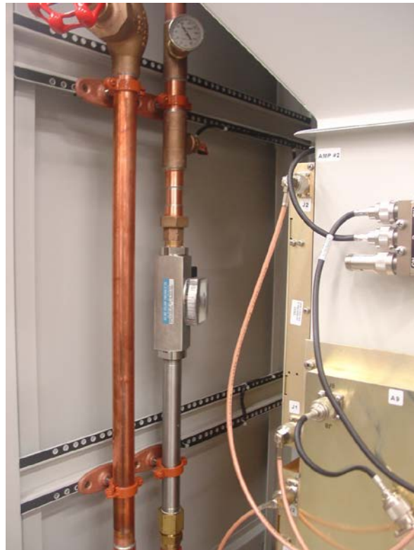
New Flow Monitor
