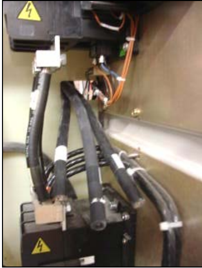
1/0 wires from newly assembled panel threaded to rear of HPA cabinet.
