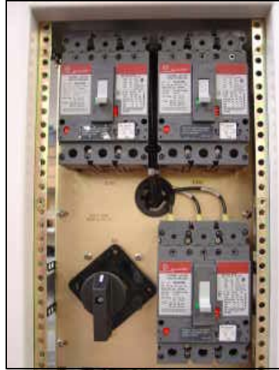
Line wires connected to CB1, CB2, CB9.
