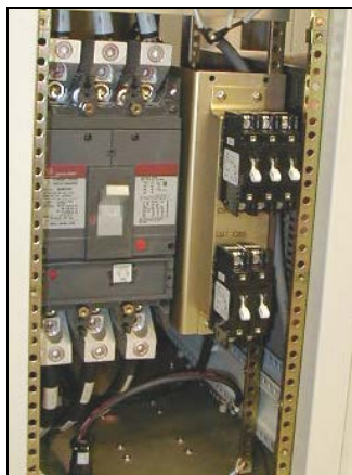
New CB3 installed.
