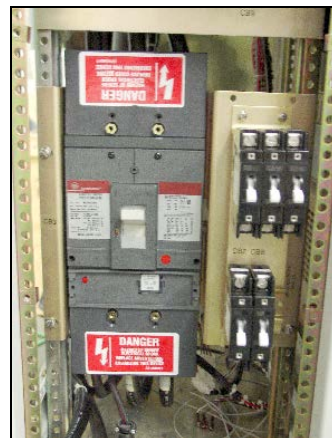
CB3 terminal covers installed.
