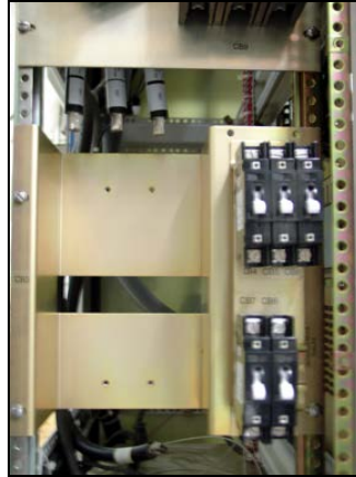
CB3/CB8 bracket installed.
