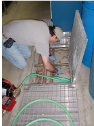
Additional drain points in floor
