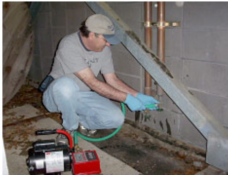
Connect to drain valve
