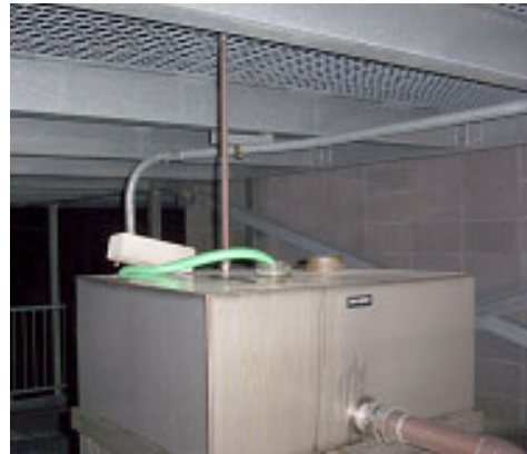
Route exhaust hose to sump tank
