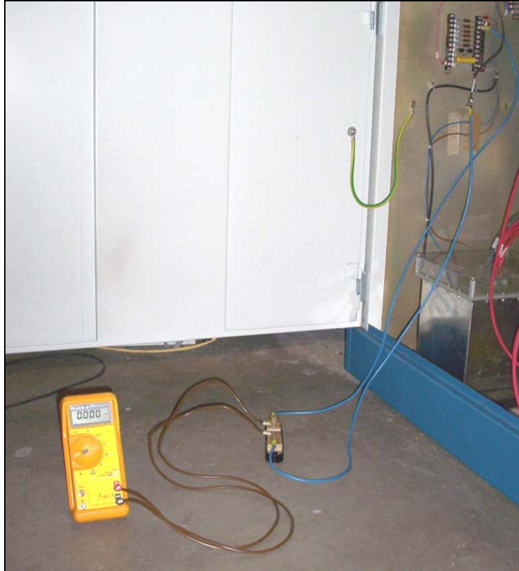
Exploded view of current shunt connections. TB11 is at upper right of photo.
